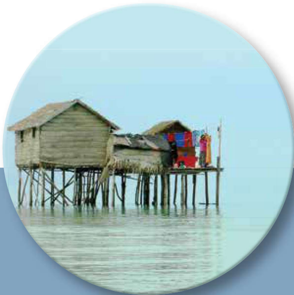
Stilt houses, Pulau Sibuan, Sabah, Malaysia
