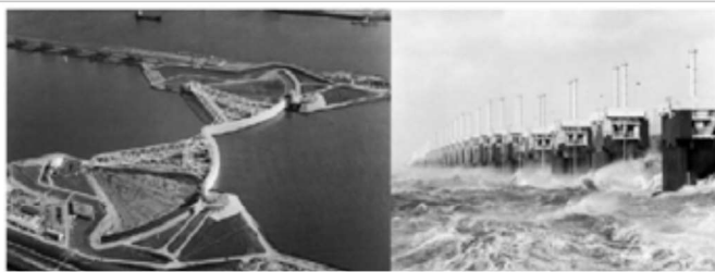
Figure 4. Maeslant storm surge barrier (near Rotterdam) and the Eastern Scheldt barrier (Rijkswaterstaat, 2009 and Jonkman et al., 2013)
